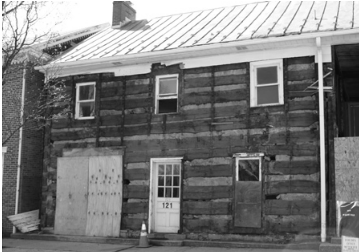
For a brief time, residents of Emmitsburg were treated to a rare view into the town's past. The exposed logs formed one of the original houses in town. Built in 1786, it was one of the few to escape the great fire of 1863.
