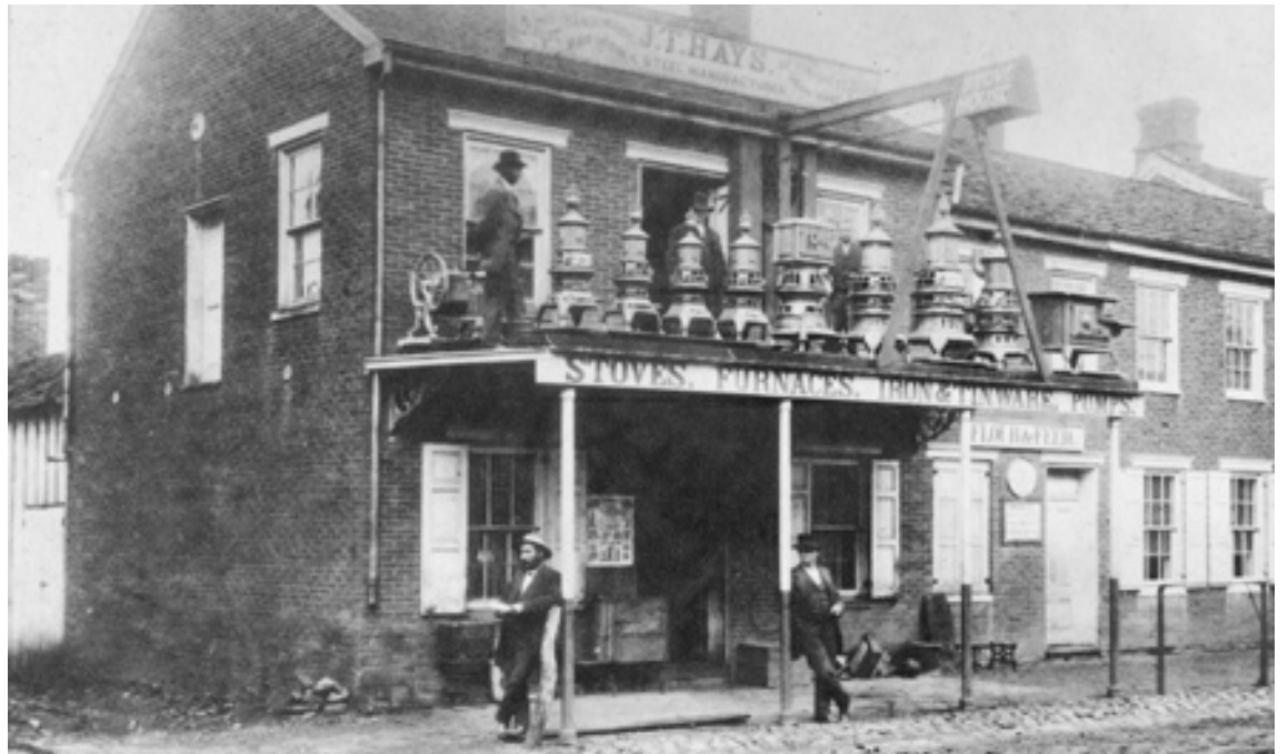
J.T. Hays Foundry on West Main St. (Photo taken approx. 1880)
