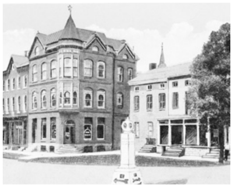
At one time the Banking House of Anna-Horner was the most eye-catching & prestigious building on the square. Fitting for the leading role it played in the development of Emmitsburg in the early 1900s.
